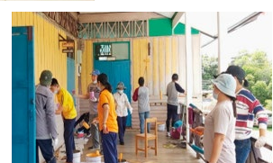
Cleaning and refurbishment of school equipment (Shindengen Thailand)
